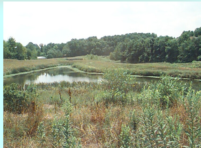
Wheaton Branch Stormwater Management Pond in Montgomery County
