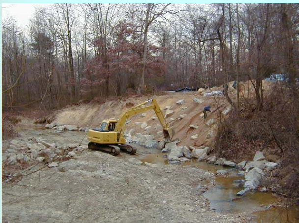
Little Paint Br. Restoration - Beltsville
