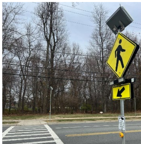
Figure 14. Rectangular Rapid-Flashing Beacon on Mannakee Street/Parking Lot 13 Entrance
