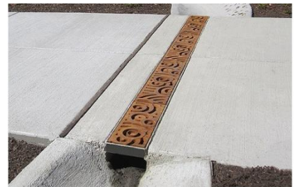
Figure 15: example of channel drain under sidewalk
