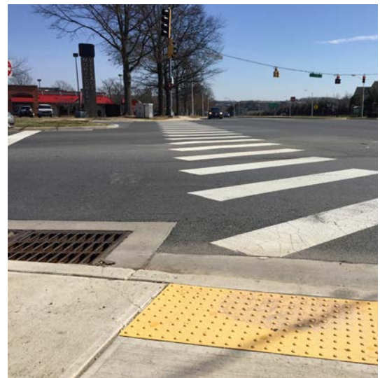
Existing northern leg crosswalk
