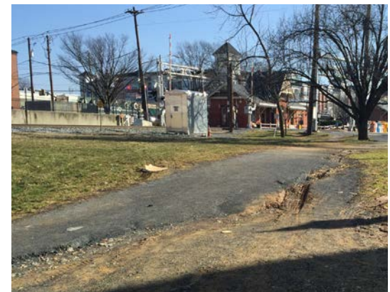
Eroded gravel path connecting the City parking garage to South Summit Avenue
