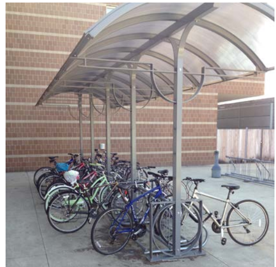
Covered bicycle parking
