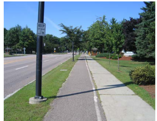
Burlington, VT sidewalk-level separated bike lane example
