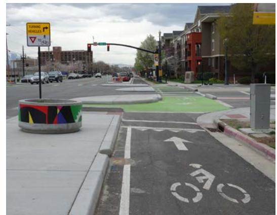
Salt Lake City, UT Protected Intersection approach
