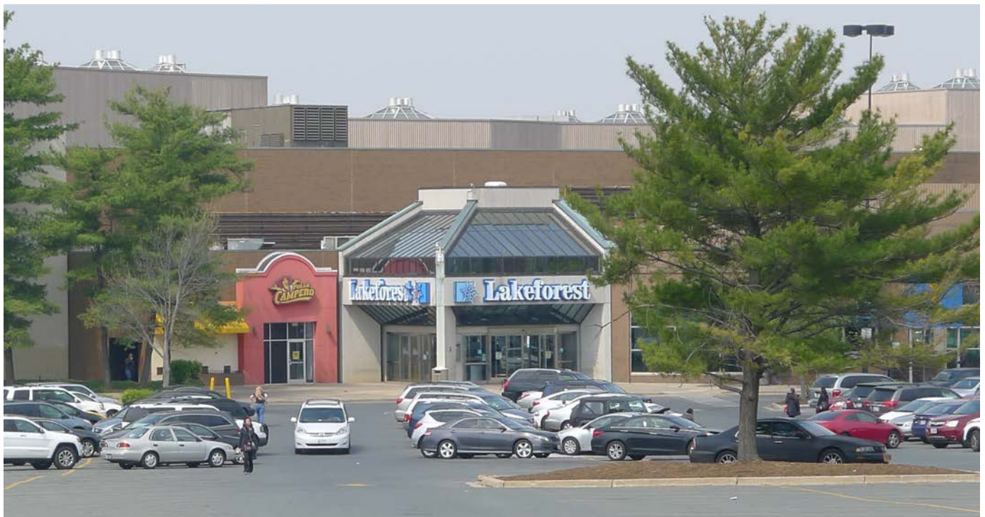
Lakeforest Mall entrance across parking lot from transit center
