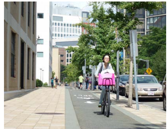
Cambridge, MA sidewalk-level separated bike lane example
