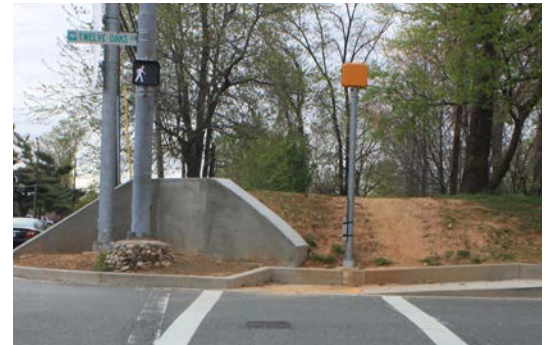
Twelve Oaks: Install a stairway along desire line to stop erosion and provide direct pedestrian travel
