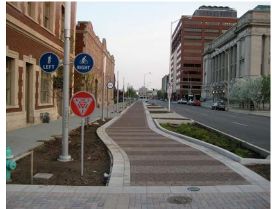
Indianapolis, IN sidewalk-level separated bike lane example
