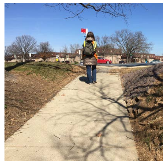
Steep slope on sidewalk connecting the Mall to Contour Road crosswalk
