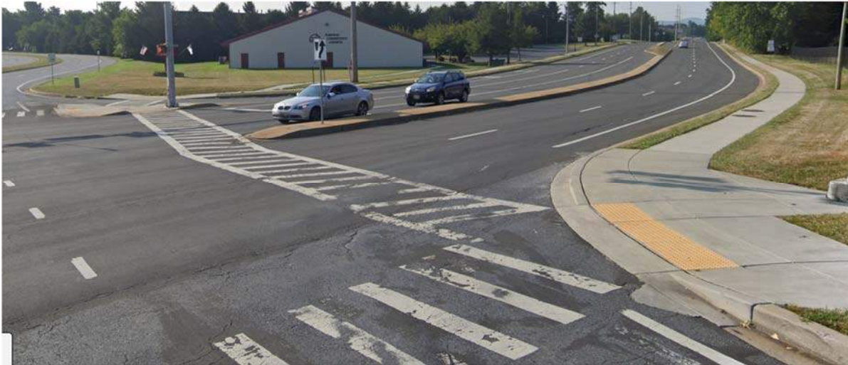
Figure 16. View of the southern leg of the Crestwood/New Design Road intersection, with a single curb ramp on the southwestern corner of the intersection and a skewed crosswalk
