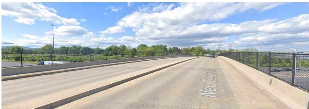
Figure 15. View of New Design Road Bridge over I-70
