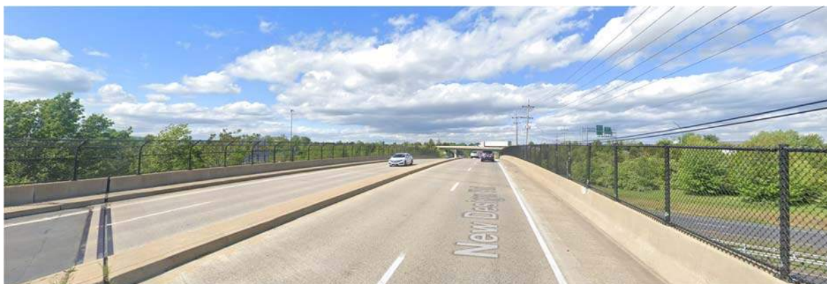
Figure 12. View of New Design Road Bridge over I-270
