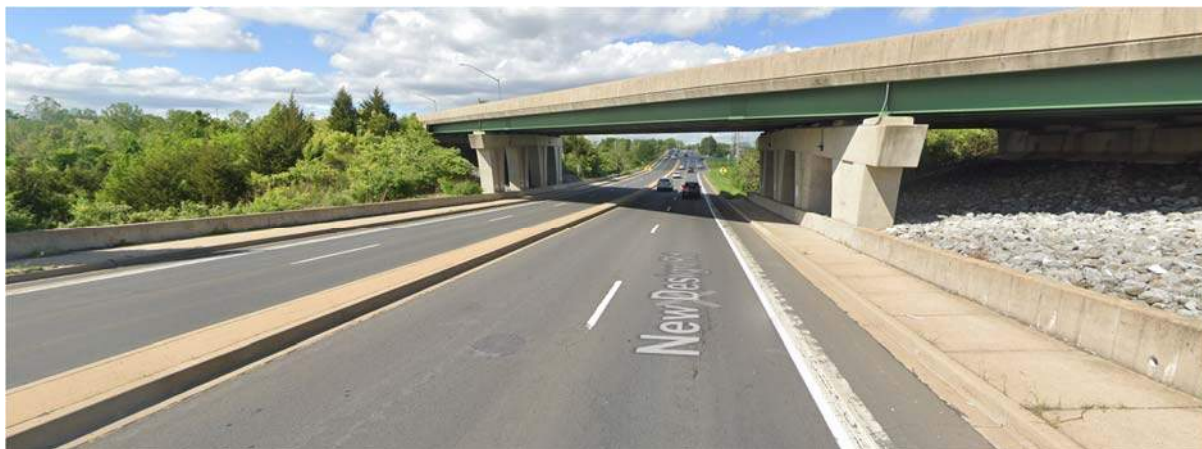
Figure 13. View of New Design Road underpass under ramp
