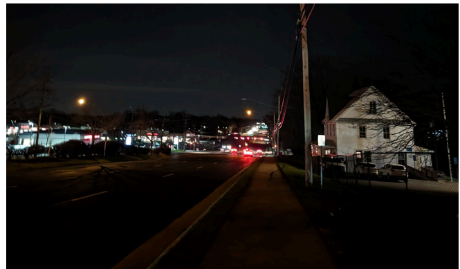
Figure 46. Dark sidewalk on south curb of Main Street between Pickett Road and Fair City Mall Shopping Center Driveway (in front of Woodson High School)
