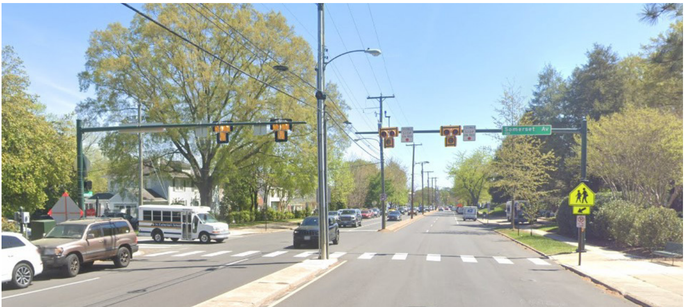
Figure 51. PHB at Grove Avenue at Somerset Avenue in Richmond, Virginia (Source: Google Street View)
