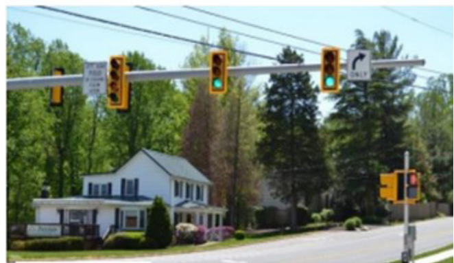
Figure 59. An Example of a High Visibility Backplates in Virginia
