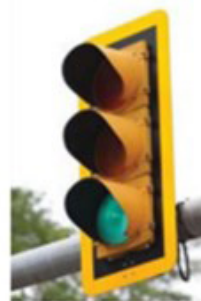
High visibility signal backplates in Virginia.
