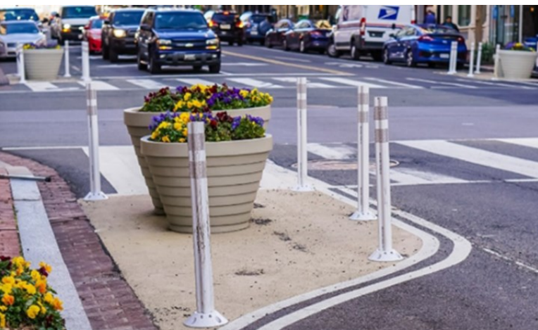
Figure 22 Temporary Flex Post Curb Extension in Washington, D.C.
