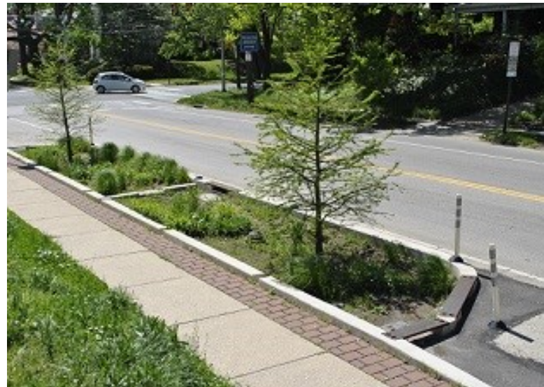
Figure 26 Stormwater Bump Out in Philadelphia, PA
