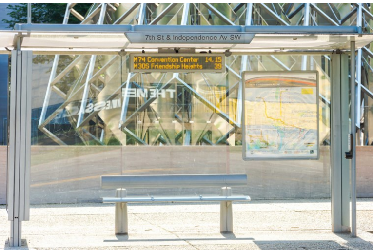
Figure 16 Bus shelter on Independence Avenue SW and 7 th Street SW
