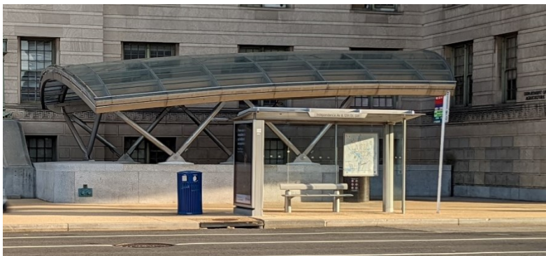
Figure 47 Transit Shelter and Metrorail Access at Independence Avenue and 12th Street SW
