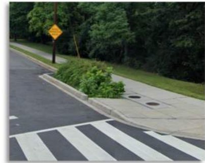
Figure 17 - SWM Facility at Curb Extension
