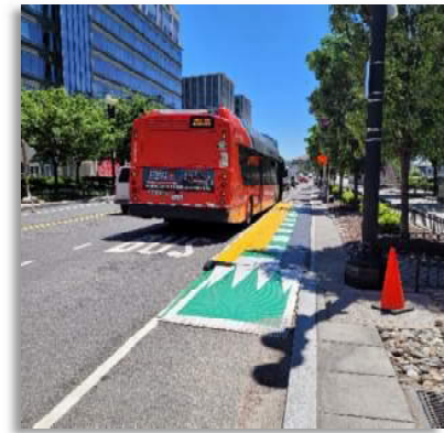
Figure 16 - Raised Bike Lane at Bus Stop
