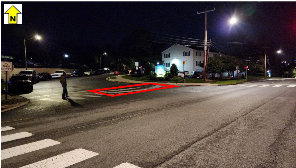
Figure 13. Example of Crosswalk Area with Insufficient Lighting (Measured vs. Visually Observed).
