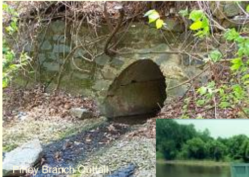
Piney Branch Outfall
