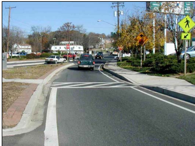
Figure 15: Slip Lane with Crosswalk ahead of Stop Sign
